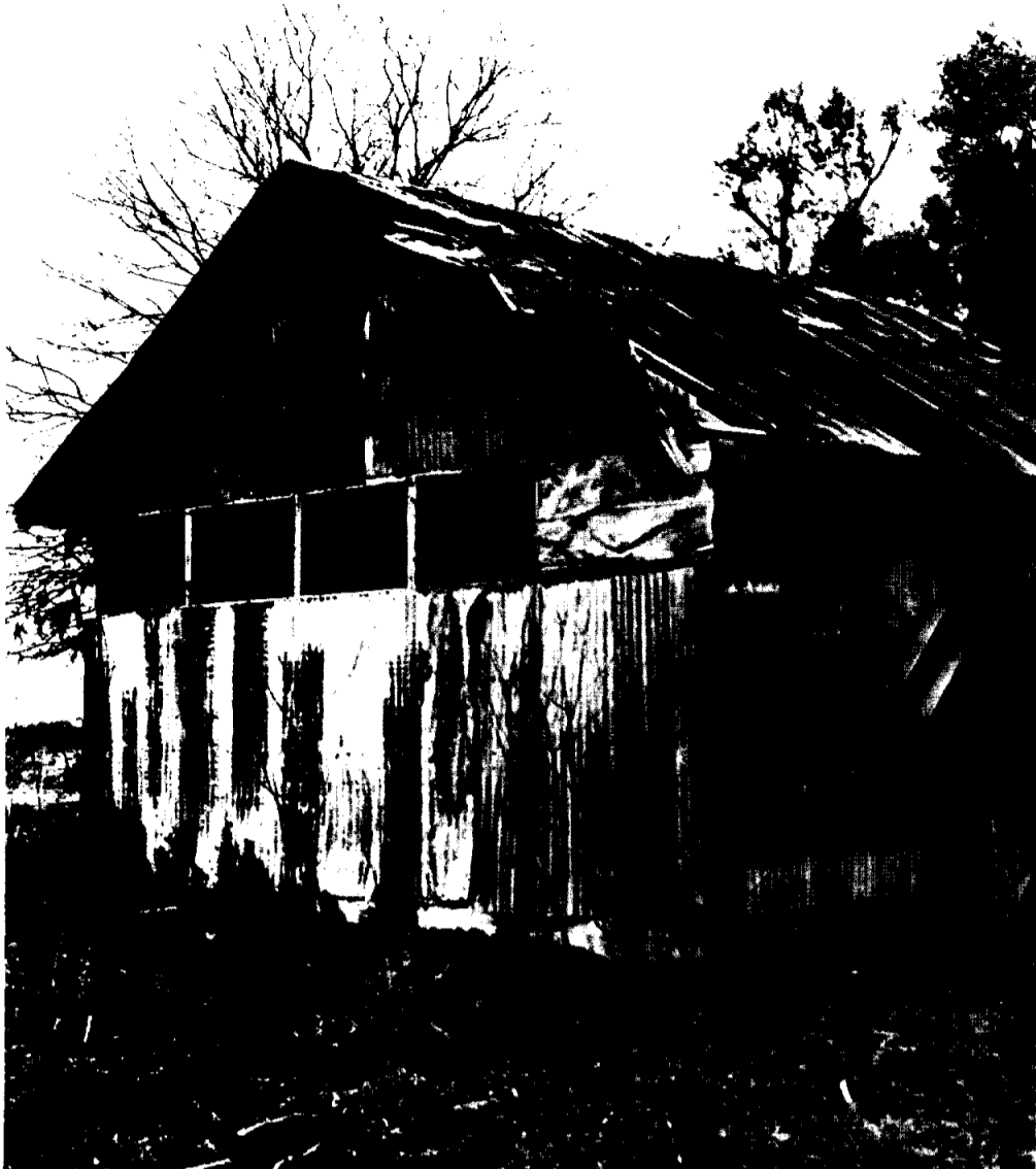
AN ABANDONED SHACK , its door inviting an errant wind to the emptiness inside, sheds shabby patches of corrugated tin onto the surrounding weeds and dreams of better days, when an old ear will give way to a new.
