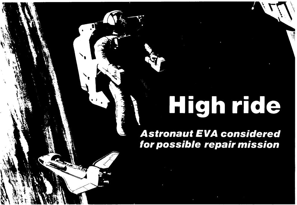
artist's conception of the traverse from orbiter to satellite during a repair mission illustrates the independence afforded astronauts with the Manned Maneuvering Unit. No tethers to the orbiter would be required, and the extravehicular activity could last for up to six hours.
