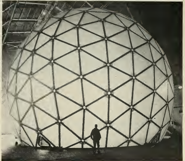
"WORLD'S LARGEST" fiberglass radome designed and built by Goodyear Aircraft Corp. for the Missile Detection Systems Section of GE, measures 68 feet in diameter and stands more than seven stories high. It can be erected by six men in 80 hours.
