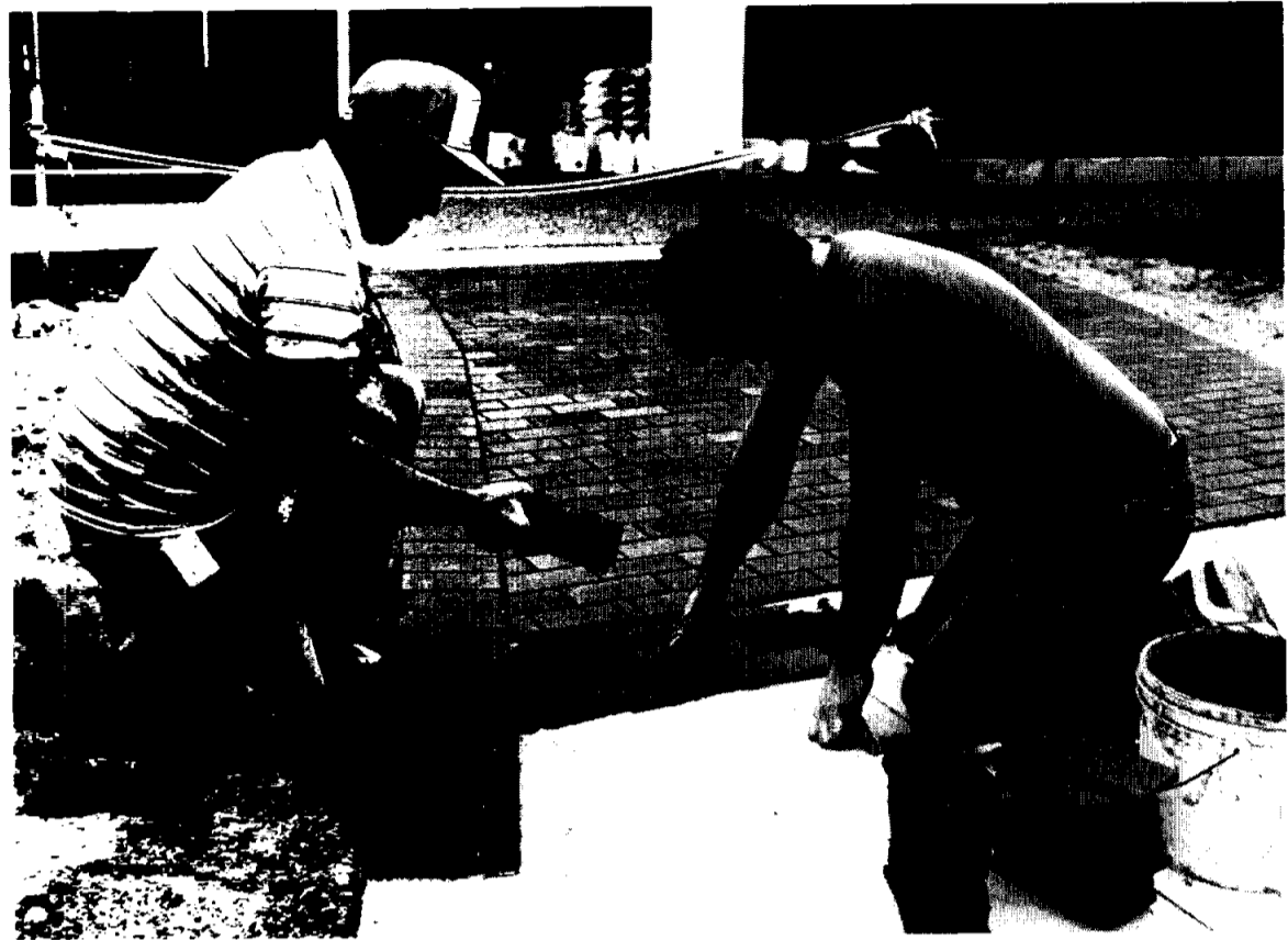
SIDEWALK DIVERSION —A father-and-son team of sidewalk pavers—Raymond West Sr., left, and Raymond West Jr.—lays half-inch quarry tile outside JSC's Bldg. 2. The new sidewalk is designed to divert public visitors on their way to the Bldg. 3 cafeteria away from the heavily traveled sidewalk north of Bldg. 1. The Wests work for American Marble, a subcontractor of Alpha Construction, the primary contractor.
