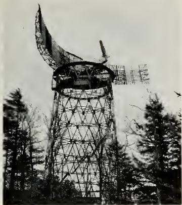
D. S. KENNEDY & Co.'s 120 ft. reflector swings continuously in azimuth at speeds up to six rpm.
