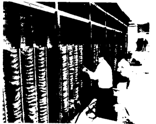
Wiring the computer termination cabinet, Bldg. 30.
