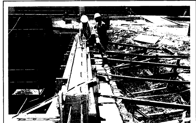
CONCRETE PROGRESS —The pouring of the foundation for the Bldg. 28 Auxiliary Chiller Facility is under way and work proceeds on schedule for completion by July 1990. Harrop Construction is building the 8,400-square-foot facility, which will provide 4,000 additional tons of chilled water to the 14,000 tons currently available to cool JSC.
