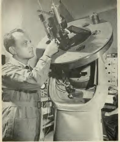
Engineer installs an air-bearing gyro on sensitive equatorial test stand in FICo test lab.
