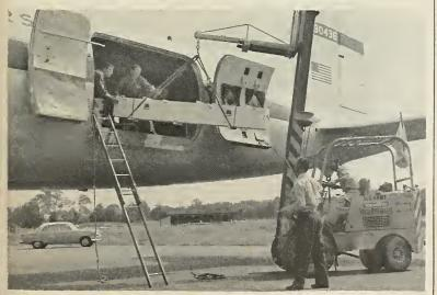
Unimpressive beginning for a very dramatic event. Thiokol RECRUIT rockets are loaded aboard a DC-7 for shipment to Eniwetok Atoll in the Marshall Islands where they will be staged as FAR SIDE vehicles. Six launchings will be made before first phase of the program is completed. Aeronutronics Systems, Inc., and AFOSR are conducting the tests.
