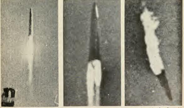
Good news for the IRBM program—Air Force THOR leaves pad in first successful flight. Taper of body and small fins can be seen.
