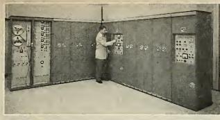
30-channel, analog-digital converter connecting 300-amplifier analog computer to 1103A digital computer
