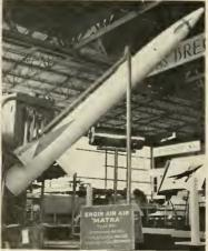
SS 10 (above left) and SS 11 (left) are surface-to-surface antitank, antiemplacement missiles powered by a solid rocket motor. Missiles are controlled by transmitting signals through two wires which unwind from a drum. The MATRA 510 (above) is an air-toair missile powered by a two-stage solid rocket motor. Missile carrier is the TRIDENT.
