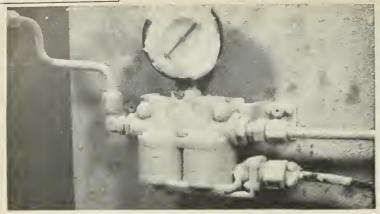
**FREEZE-UP** of solenoid controlled valve in airborne system at  $-65^{\circ}$ F can choke off vital air supply. Manufacturer faces tight contract delivery schedule.
