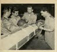
Officers of the Italian Air Force probe the "insides" of a NIKE-AJAX surface-to-air during a class in repair and maintenance.
