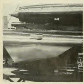
A close-up view of the double-wedge five per cent airfoil hinged wing attachment, booster slipper bracket and front of THOR ramjet.
