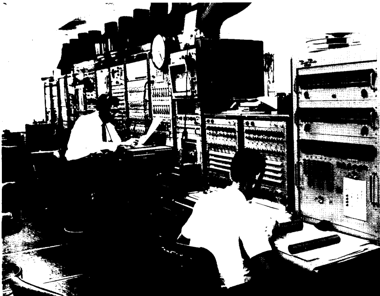
A PORTION OF the intricate equipment which plays an important role in the overall operation of the Mercury Control Center.
