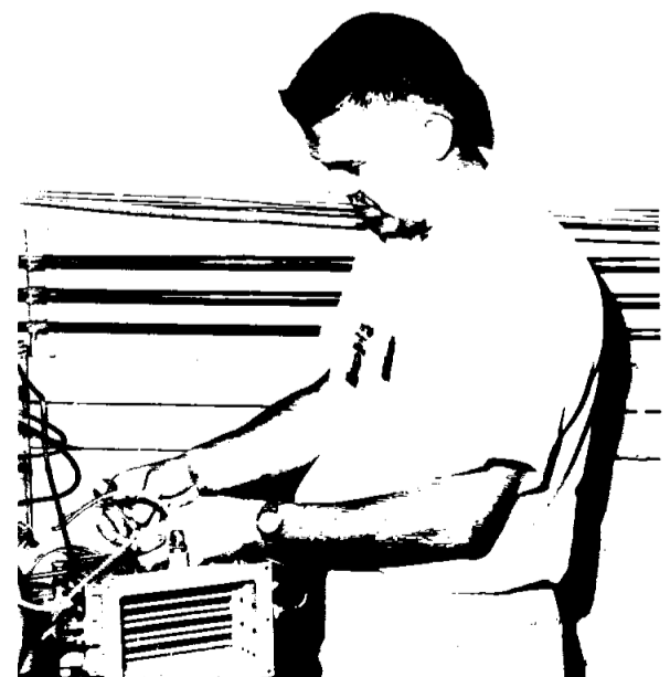
PAUL O. FERGUSON , of the Instrumentation and Test Section, Crew Systems Division, works on a Gemini cabin heat exchanger.
