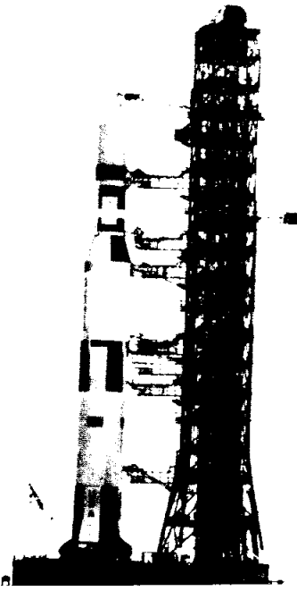
SKYLAB I AND II ON PAD—A deliberate double expose to help illustrate the comparative sizes and configurations of the Skylab I and II space vehicles at Launch Complex 39, Kennedy Space Center, Florida. The double exposure creates an illusion that the rockets are side by side, though actually they are 1½ miles apart. The Skylab I/Saturn V space vehicle is on the left. On the right is the Skylab II/Saturn 1B space vehicle.
