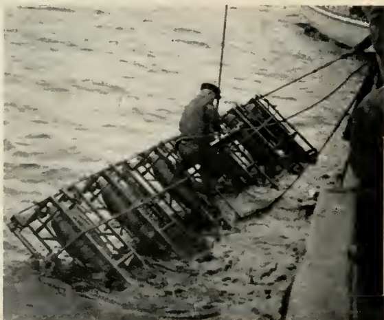
Collapsible launching gear for solid rockets being installed on W-class long-range sub. Rack holds six missiles.
