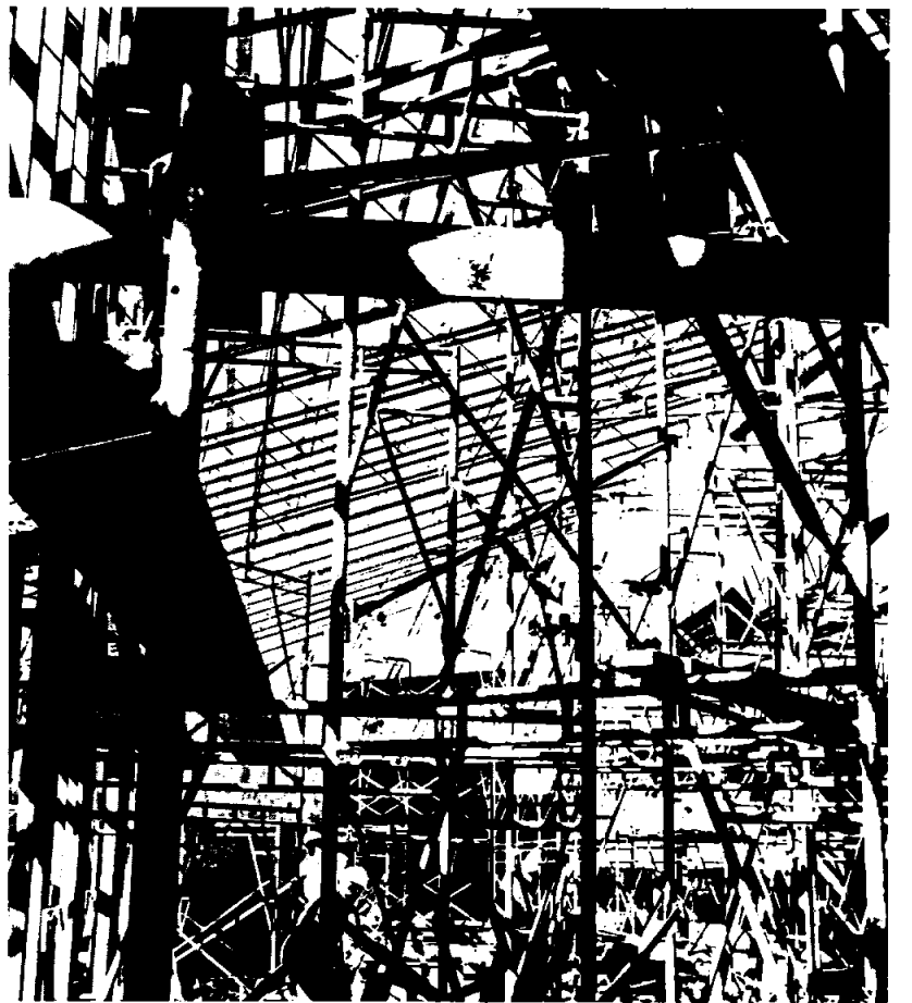
CREDIT UNION—Construction is now well underway for the new JSC Credit Union Building which is expected to be completed in February of 1975. The building is located across from the back JSC entrance on Gemini and Saturn.
