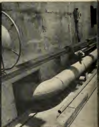
Fuel lines and process piping are Stainless Steel and operate at pressures up to 15,000 psi. The pipes are kept almost surgically clean to prevent contamination of fuel and subsequent malfunction. Vapor degreasing and chemical cleaning processes are used on the pipe.
