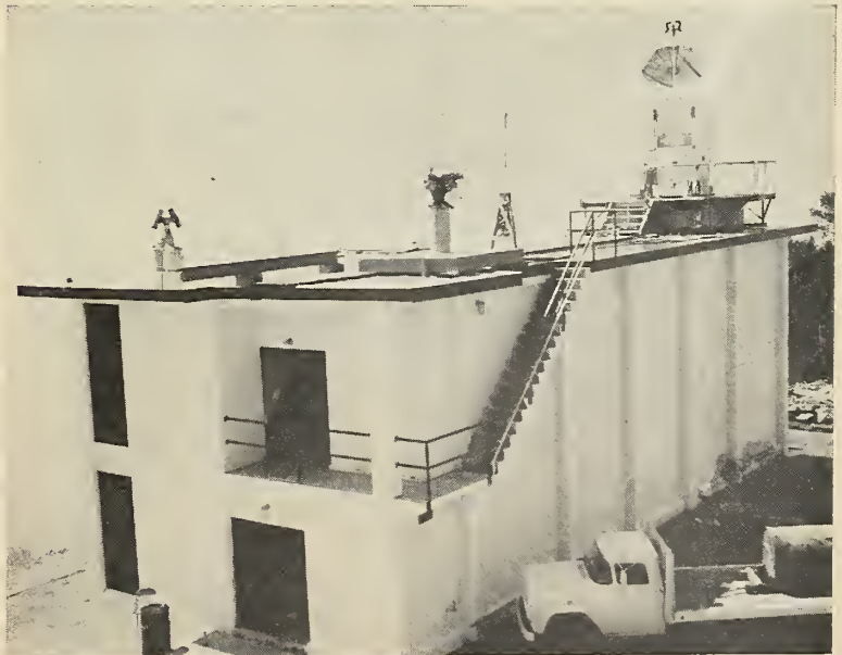
TRACKING RADAR building on top of 21,500-foot Mt. Tranquillon houses newest long-range radars and other tracking instrumentation for PMR.
