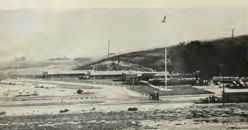
ADMINISTRATION BUILDING and related facilities near completion at Point Arguello. The 20,000-acre Point is the heart of the would-be $4-billion Pacific Missile Range.
