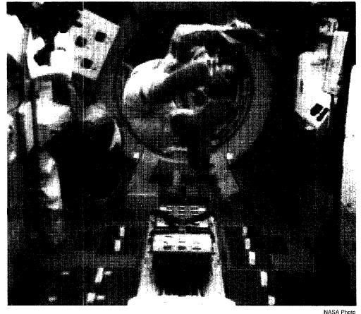
STS-42 Payload Specialist Roberta Bondar floats above the International Microgravity Laboratory's sled device during Spacelab activation. The sled is being used as part of the Space Adaptation Syndrome Experiments, measuring changes in the otolith organs that provide humans with a sense of up and down.
