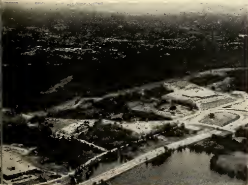
WALTHAM Research & Development Park. Thirteen industrial buildings are either finished or in final construction stages.
