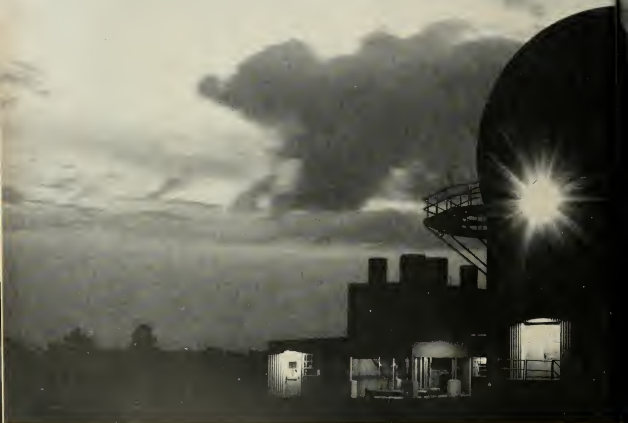
Westinghouse AN/FPS-27 Radar in operation at an Air Defense Command site
