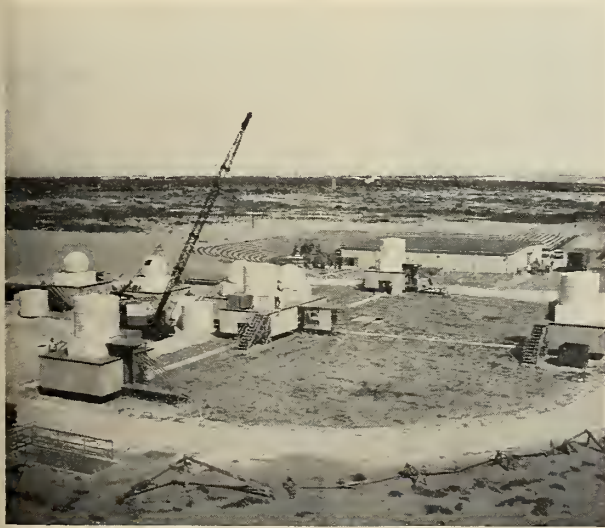
TEN ANTENNAS and necessary support equipment comprise the new Azusa Mark II tracking system built for the Air Force by Convair. The system can detect flight positions of up to one-tenth foot.
