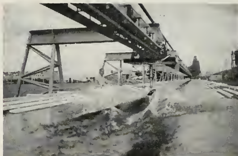
New $300,000 Convair San Diego seaplane towing tank, first unit of complete hydrodynamics laboratory.
