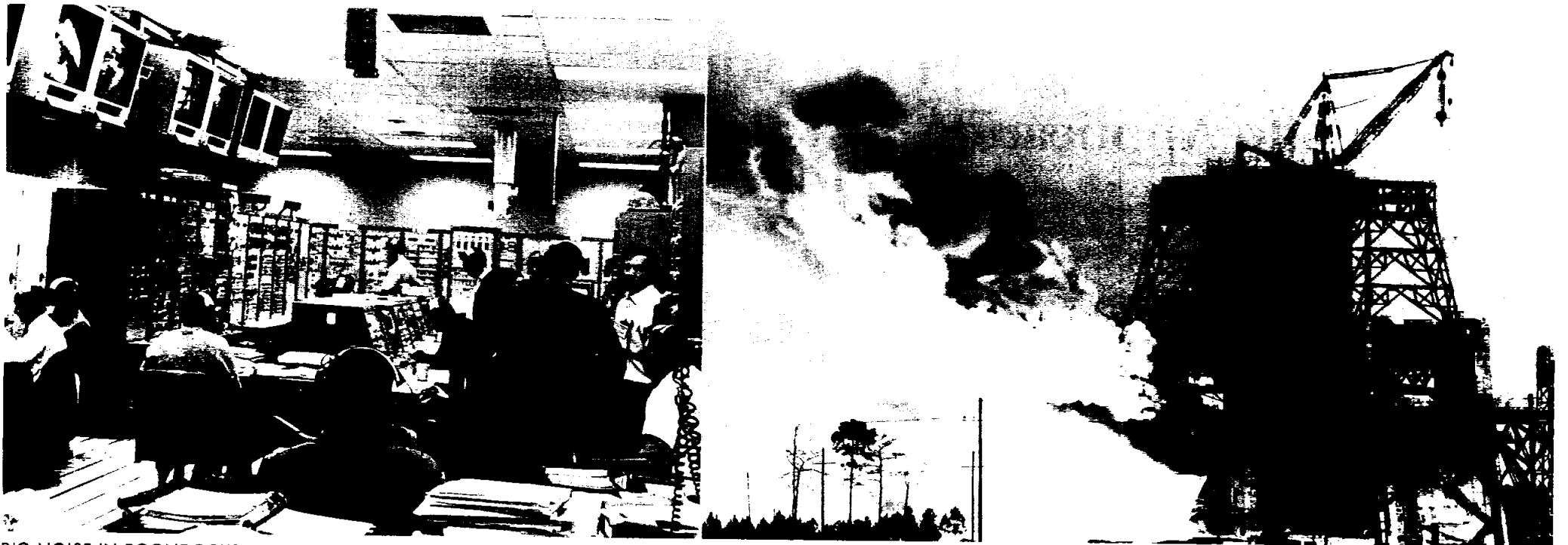
BIG NOISE IN BOONDOCKS —Test engineers in the S-IC test stand control room, left, monitor systems displays during the countdown for the March 3 static firing of a Saturn V first stage test article. At right, many decibels of noise rumble out across the southern Mississippi
