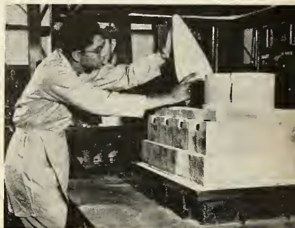
TECHNICIAN PLACES radome in bottom of the kiln preparatory to firing.
