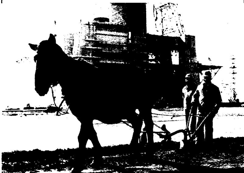
FORGOTTEN BUT NOT GONE —One mulepower was found to be the best way to dig shallow trenches for piping near the Saturn V static test stand at Mississippi Test Facility where S-IC stages develop the equivalent of 160 million horsepower.
