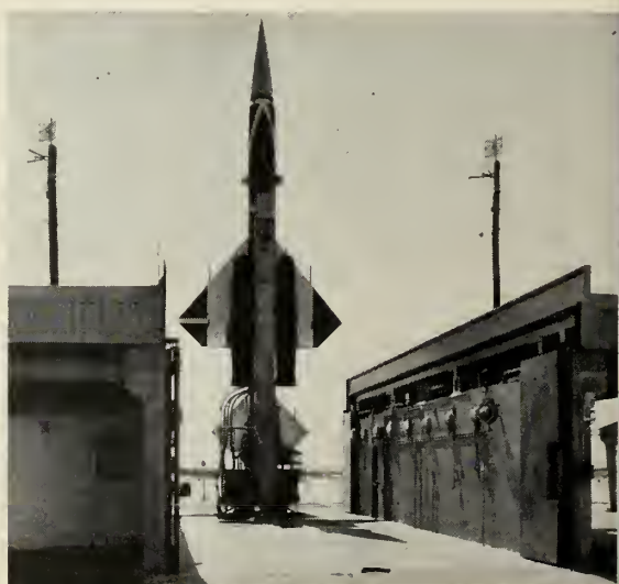
MATERIEL REQUIREMENTS were cut sharply in this Model II shelter now operational at McGuire AFB, N.J. The structure is steel.
