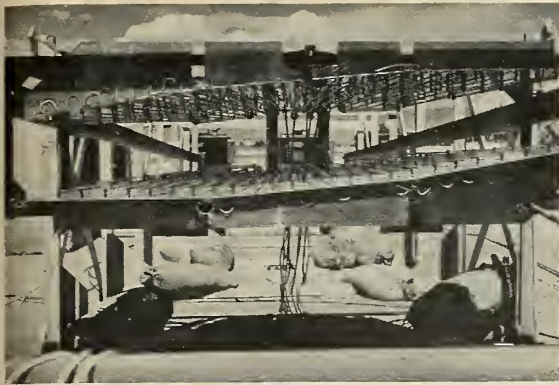
PRIOR TO run start, each fin was heated to approximately 600°F by GE-T3 quartz heating lamps to simulate aerodynamic heating since such heating would not occur during short duration of test. Lamp reflectors, originally used in fin static tests, were modified by Narmco, which also designed reflector carriages and withdrawal track to pull heater panels back prior to sled start. Lamps were re-spaced in reflectors for correct maximum temperature distribution with constant power input to eliminate complex and elaborate temperature controllers.
