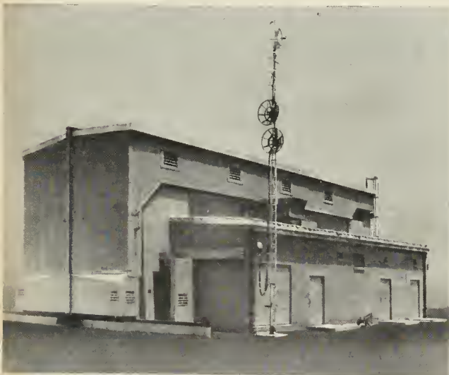
EVOLUTION OF Bomarc launching shelters began with this prototype Model I. The building required nearly 1000 tons of concrete.
