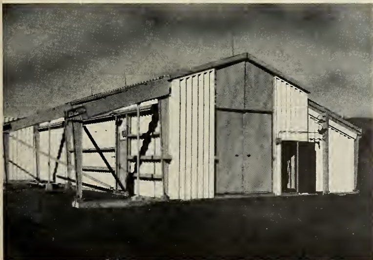
THIS IS THE ONLY Model III shelter yet built. While cheaper than Model II, this type proved to be "ultimate in complexity," so Air Force quickly dropped it.
