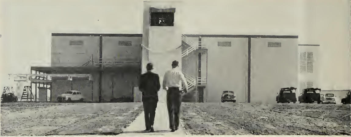
THIS PRIMARY TOWER in "boresight range" is one of two tall structures at Ryan's newly opened facility which are important in microwave study. Transmitting tower stands on a concrete base 15 ft. above ground with about 38 ft. underground.
