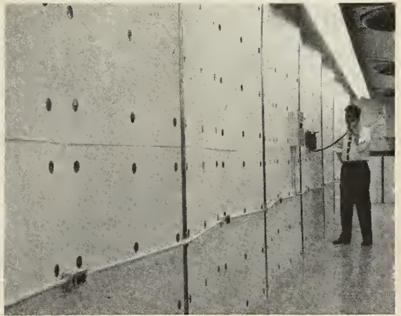
IRREGULAR SHAPE of wall and ceiling helps reduce noise in vibration test facility. Acoustical materials bring sound level down from 120 decibels at source to 45 decibels, equal to a radio's hum.
