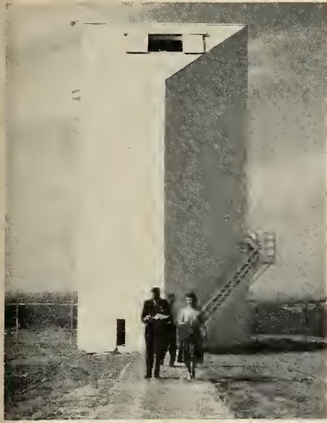
SECONDARY tower has antenna dish to return transmitter tower's signal. Odd building design prevents signal bounce back from surfaces other than dish.
