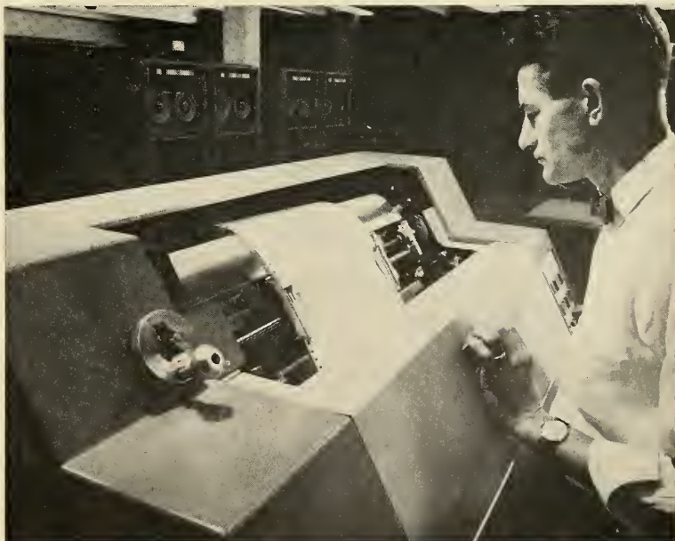
900 LINES a minute is the speed of the printer included in the Minneapolis-Honeywell Regulator Co. 400 high-speed electronic data processing system.
