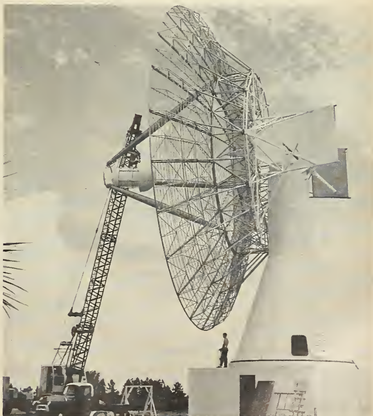
New, giant ICBM tracking antenna designed by Radiation, Inc. Unique feed system at center of the reflector gives conical scan. Antenna automatically homes on telemetered signals from the missile. Rate-memory circuit continues tracking during fadeout or noise period.
