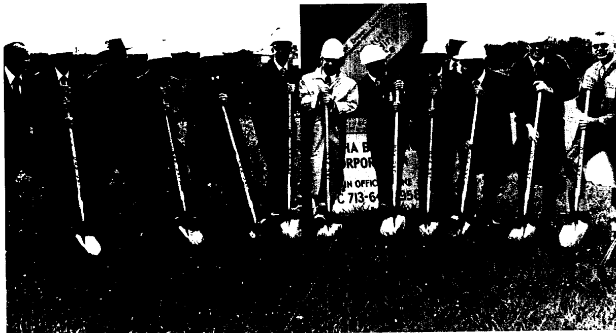
GROUND BREAKING CEREMONIES-A ground breaking ceremony was held Monday, April 15, at the site of the soon-to-be-constructed JSC Credit Union building at the corner of Gemini Boulevard and Saturn Lane. Pictured above are Credit Union Board of Directors, the building architect and contractor, and JSC director, Dr. Christopher Kraft (fifth from left) who were on hand for the ceremony. From left to right: Walter Duson, Ron Gerlach, Bill Milam, Ed Campagna, Dr. Kraft, Jerry Haptonstail, Harold Ferrese, Paul Startevant, Sherman Kendall, Gordon Kovich, Ed Stelley, Tom Drenek, James Moody.
