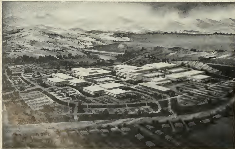
ONE OF the valley's new facilities now under construction is this group of labs for Thompson Ramo Wooldridge, at Canoga Park, designed by Albert C. Martin & Assoc.
