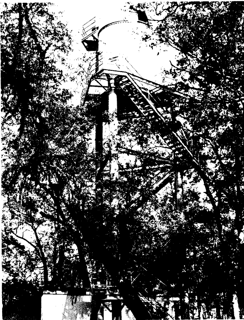
SUN WATCH — The dome of the Solar Particle Albert Network rises through the moss-draped oaks at the northeast corner of the MSC site. The spectrograph and the lower end of the heliostat and office space are housed in the building at the base of the tower.
