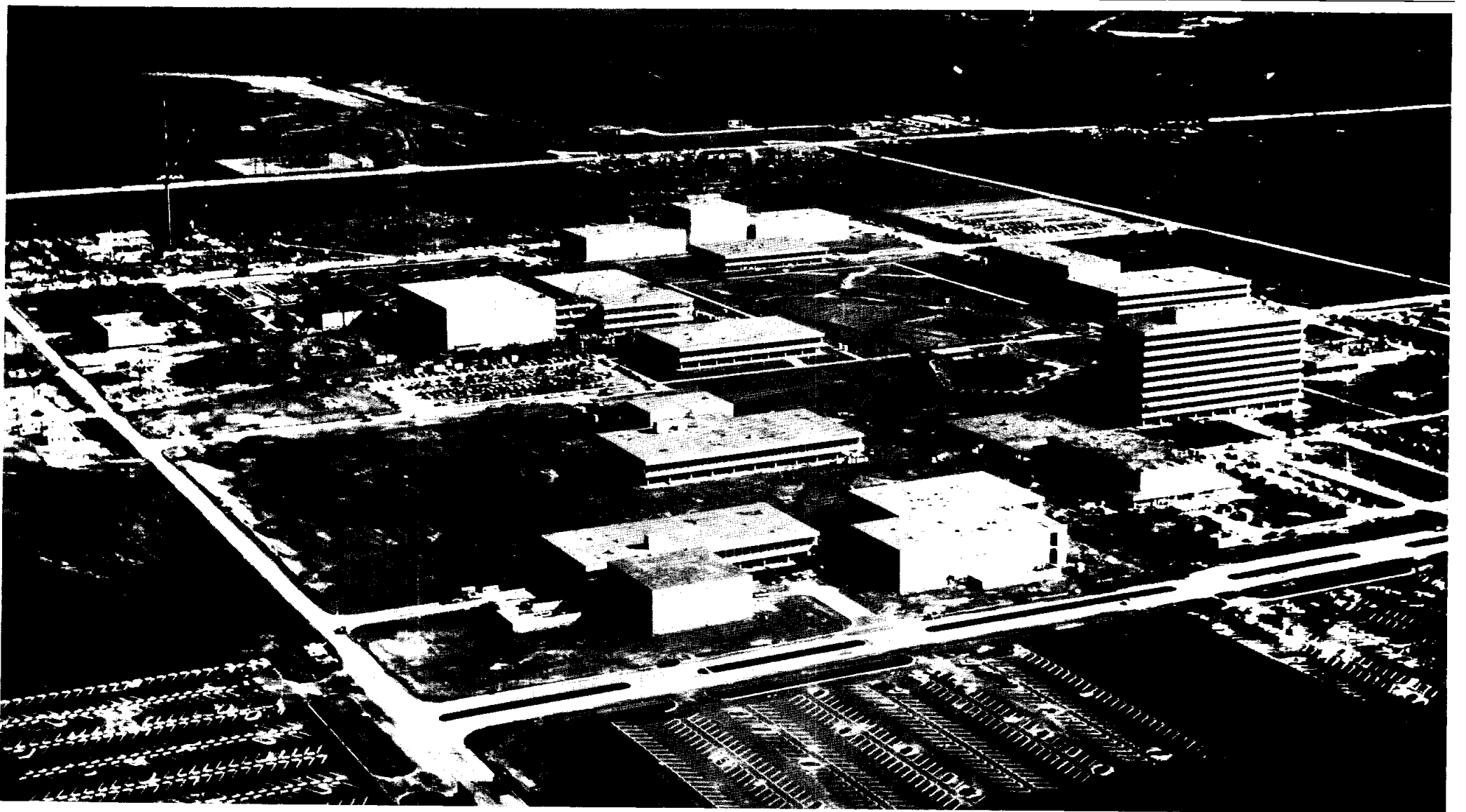
CLEAR LAKE SITE CONSTRUCTION PROGRESS -In this aerial view of the Manned Spacecraft Center, Clear Lake Site, looking northeast, construction progress is clearly visible. Beginning with the nine-story Project Management building on the right and going clockwise, the major buildings are as follows: Auditorium, Systems Evaluation, Instrumentation and Electronics, Spacecraft Research, Central Data, Mission Control Center, Technical Services offices and shops (the taller building in the rear is the shops with the offices in the building immediately to the front), Life Systems, Flight Operations, and just to the right of the Project Management building is the
