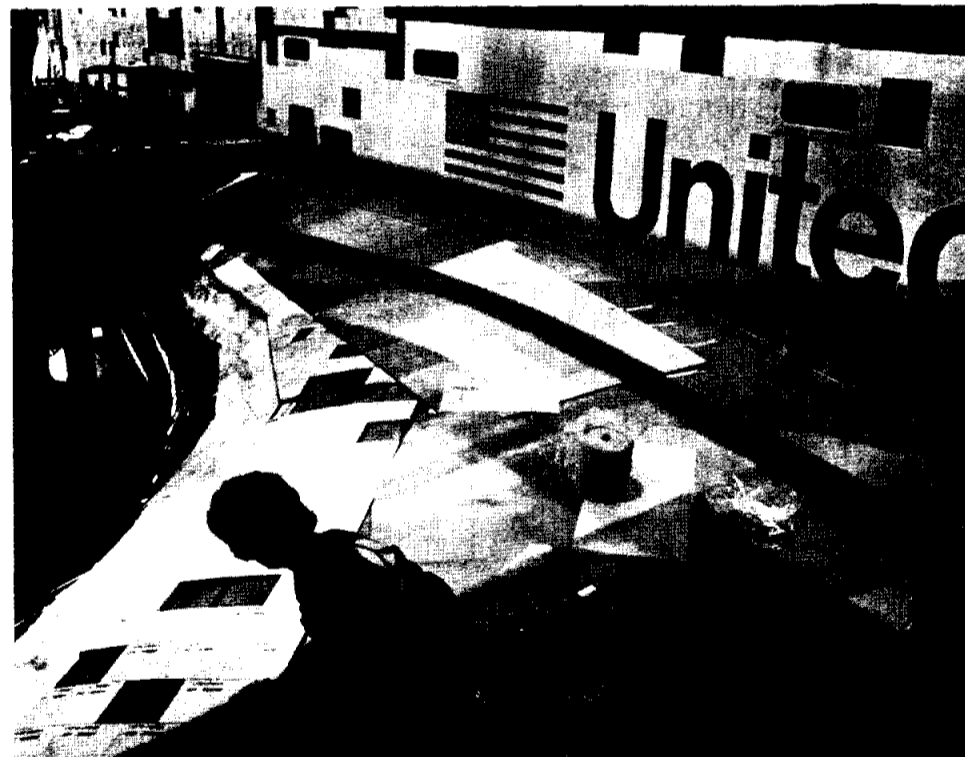
Above is tile installation in process at the Cape. The heat protective tiles are a major factor pacing the Shuttle schedule.
