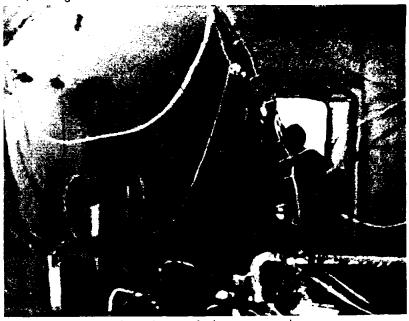
Henry Rotter enters from the man-lock as soon as the emergency repressurization reaches 27,000 feet and releases Le Blanc's suit glove clamp rings to allow oxygen to enter the suit and revive him.
