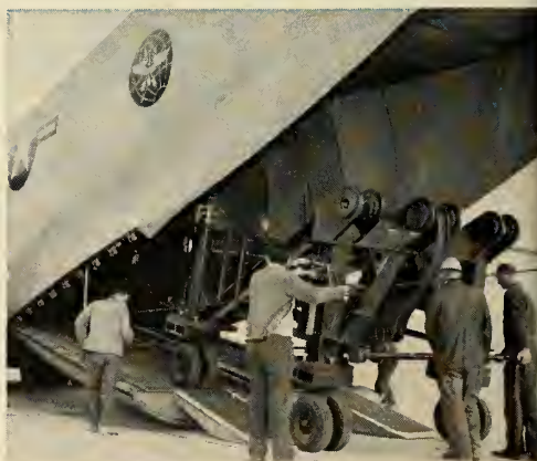
Missile equipment takes to the air in Air Force's giant C-130 transport which flew FMC-built Thor ground support equipment from West Coast to test site of Cape Canaveral, Florida. First load (upper) takes 65' launcher-erector section. Launching base and power-pack trailer (above) were flown in a second shipment.
