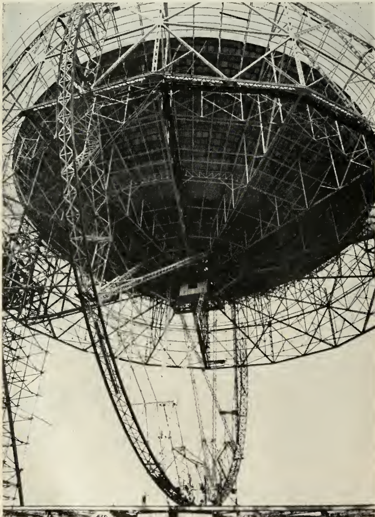
GIANT RADIO TELESCOPE in Jodrell Bank near Manchester, England, is used to provide the initial tracking lock-on for the moon probe, and is ten times larger than any other of its type. Automatically steerable, it weighs 2,000 tons and revolves on bogies laid in a circle with a diameter of 360 feet. The telescope has the capability of reaching out into space one billion light years. Scientists at Jodrell Bank have already been able to detect radio waves emanating from the nebula in Andromeda, five trillion miles from earth. Pictured is a view underneath the radio telescope showing the stabilizing wheel, the motor house on the diametral girder and, underneath, the hanging laboratory which pivots on trunnions as the bowl rotates.
