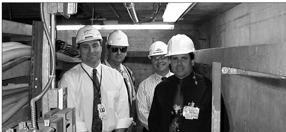
The Phase 2 Utility Tunnel Upgrade Construction Team, from left, includes Ray Burnette, Gilbane Building Co.; Jim Jones, project superintendent, C. L. Vick Construction Co. Inc.; Bob Kehoe, NASA construction manager; and Steve Campbell, project manager.
