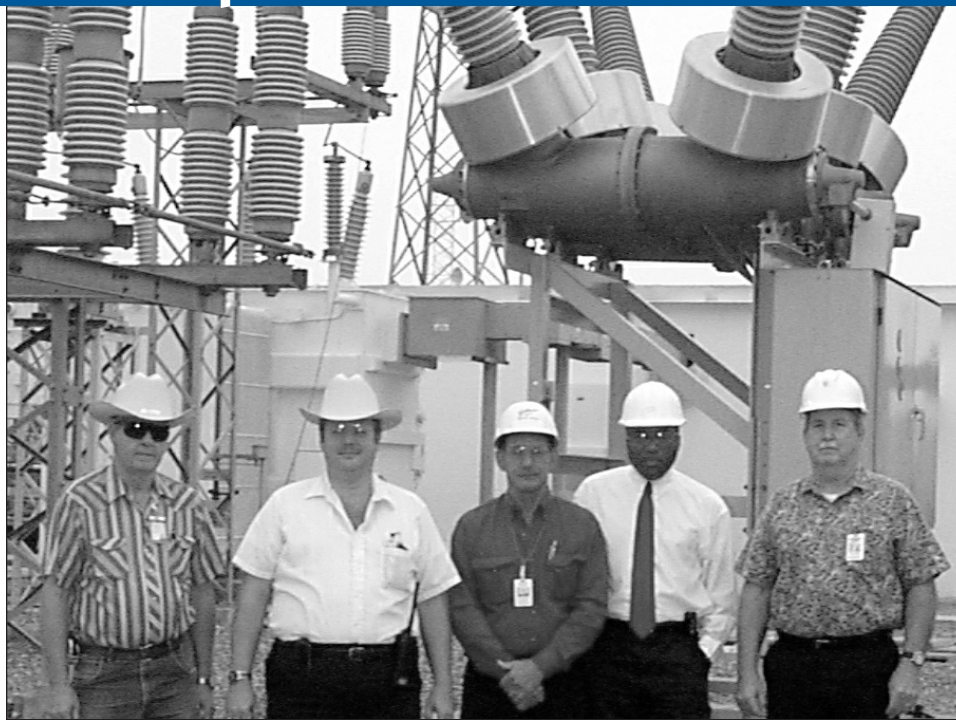
The Site Electrical Substation Construction Team, from left, includes Bill Harkleroad, project superintendent, Gardner-Zemke Construction Co.; Reinhard Brueckner; Ben Richardson, Gilbane Construction Co.; Marvin Bennett, NASA construction manager; and Bud Nichols, project engineer.
