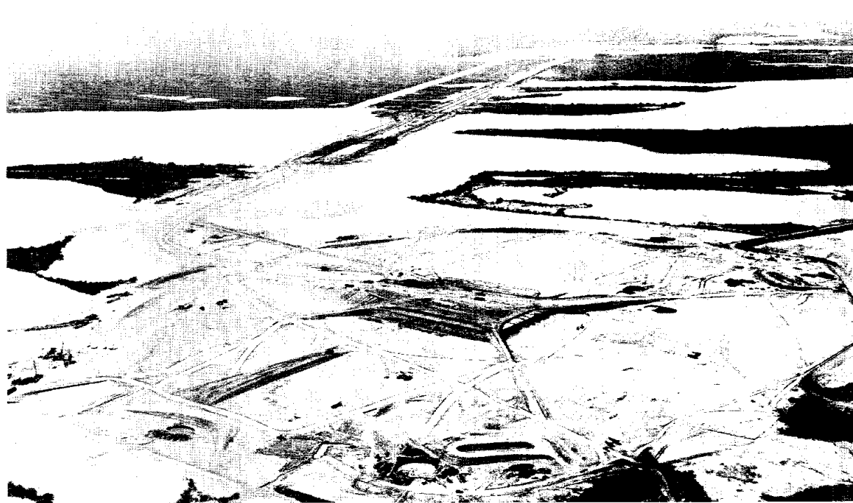
PAD 39A - This aerial view of the Merritt Island Pad 39A area shows the build up for the pad in the center of the photo. Going off the pad to the left and making a 90 degree turn to the right is the crawlerway that connects Pad 39A (Saturn V launch pad) with the Vertical Assembly Building under construction in the background.
