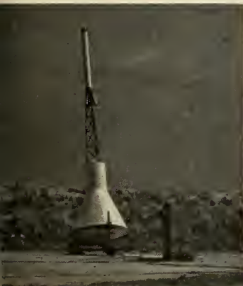
ESCAPE MECHANISM of the Project Mercury manned orbital capsule is tested at NASA's Pilotless Research Station at Wallops Island, Va. Mechanism is in the tripod arrangement on full-scale model weighing about one ton. Escape rockets lifted the capsule to 2250 feet where the tripod was ejected and a parachute lowered the capsule to the water where it was recovered by helicopter.
