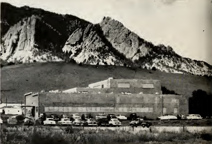
OUTSTANDING cryogenic research is being undertaken by the NBS-AEC Cryogenic Engineering Laboratory in Colorado.
