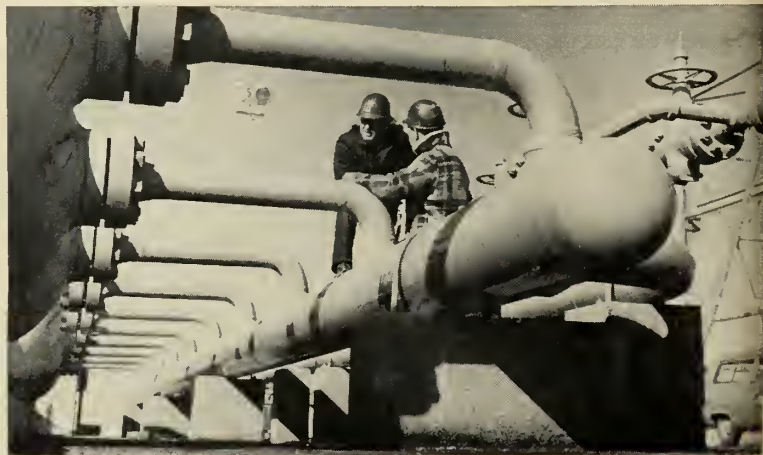
THESE HIGH-PRESSURE gas containers will be used in testing NASA's F-1, or Nova vehicle, rocket engine. Tanks service Stand 2-A at Edwards.
