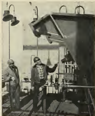
ENGINEERS inspect thrust mount for F-1 test facility.
