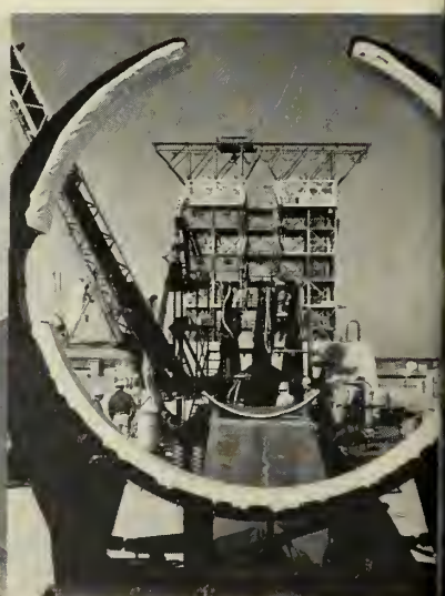
The mobile transporter for the Thor is strong but light on its wheels because it was designed with weight-saving high-strength steels. Slanting to the left is the steel umbilical tower which carries Stainless Steel fuel lines and control lines.
