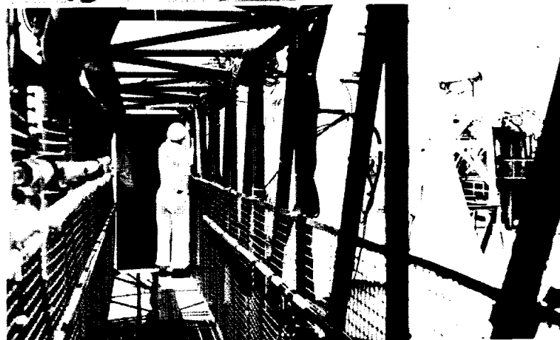
WALKWAY TO THE MOON —Access arms or walkways for Saturn V mobile launchers are thoroughly wrung out in tests at the Marshall Space Flight Center prior to shipment to Kennedy Space Center. In the top photo, a command module mockup is mounted on a motion simulator which duplicates the swaying of a Saturn V in high winds. The lower photo shows the crewman's view as he leaves the elevator and hikes across the access arm.
