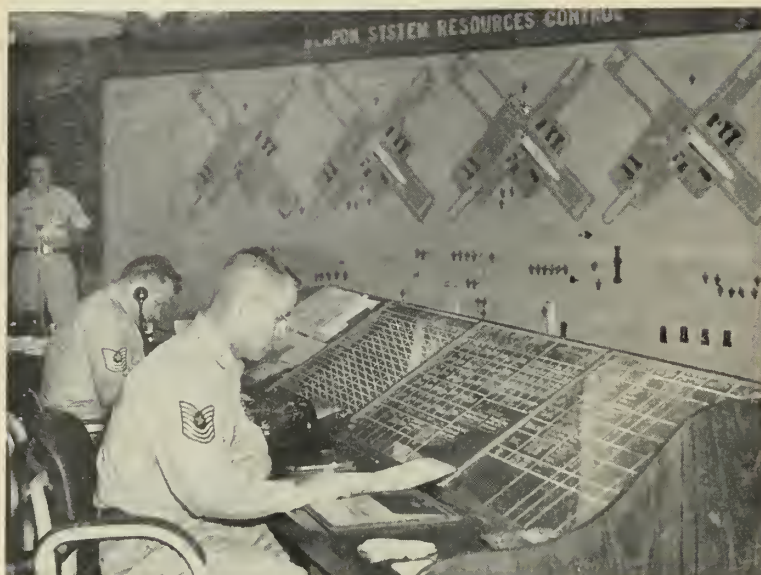
CONTROL ROOMS, such as this one built for Thor training, enable all training operations on launching pads to be followed by training directors.
