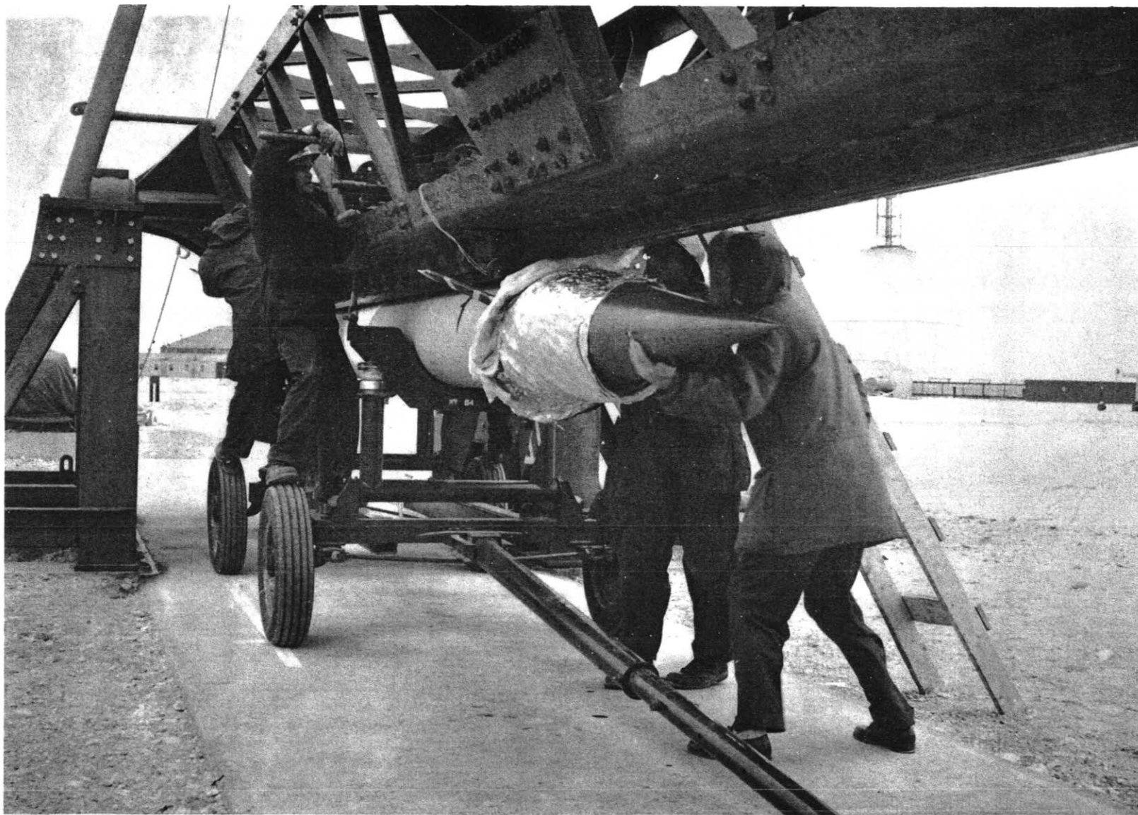
Installation of Black Brant I on the launcher.
