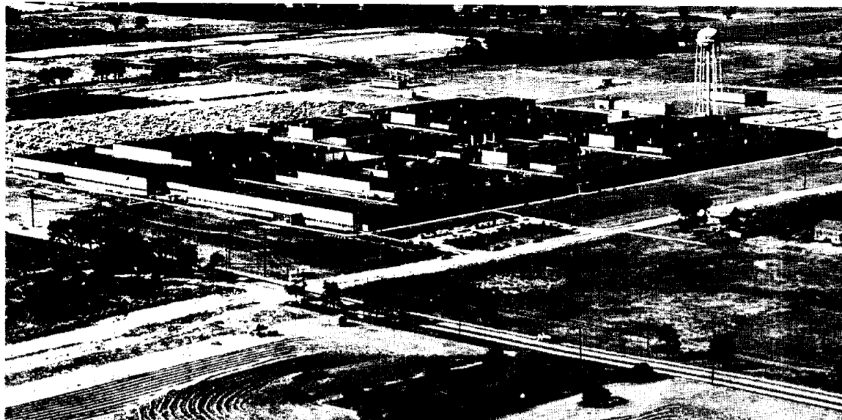
AERIAL VIEW OF AC-MILWAUKEE —This 767,000 sq. ft. facility is the largest of AC Spark Plug Division's three Milwaukee plants. Here AC will manufacture inertial guidance systems for the Apollo spacecraft.
