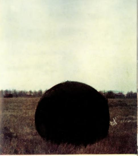
Sharik [Sphere] stood up to all the tests—the 20 ton stress, 10,000 temperature which caused it to be enveloped in flames as it passed through the dense layers of the atmosphere. The protective coating performed its function well. Incidentally Sharik is good for another flight.
