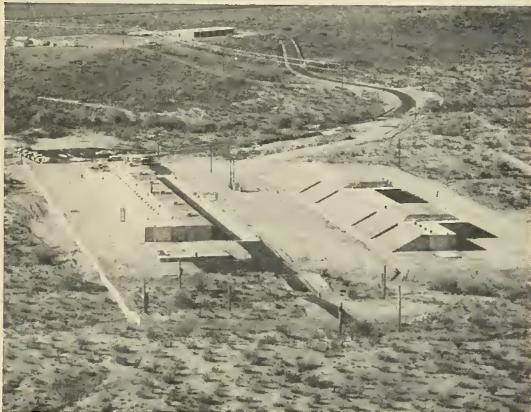
SOLID FACILITY near Mesa includes (at left) building for preparational and finishing operations, (at right) heavily barricaded structure for hazardous mixing, curing and loading, and (background) 7000-square-foot engineering building.
